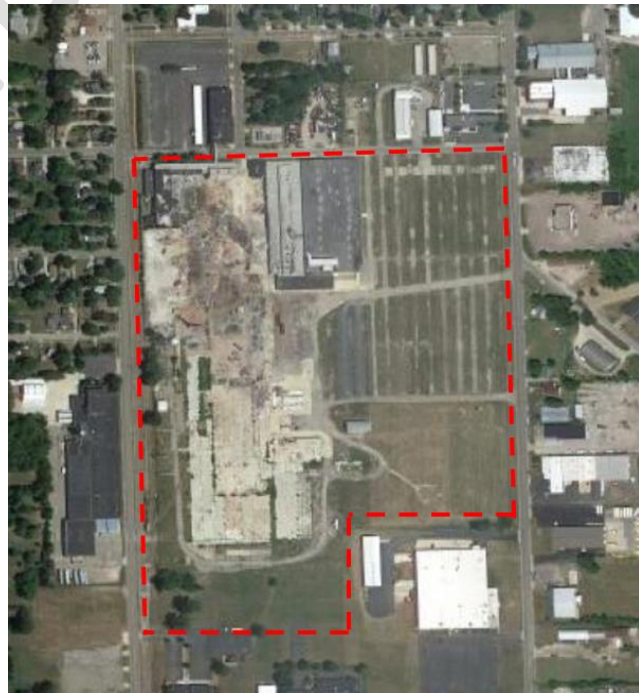
Potential Site Location
